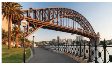
Sydney Harbour Bridge
